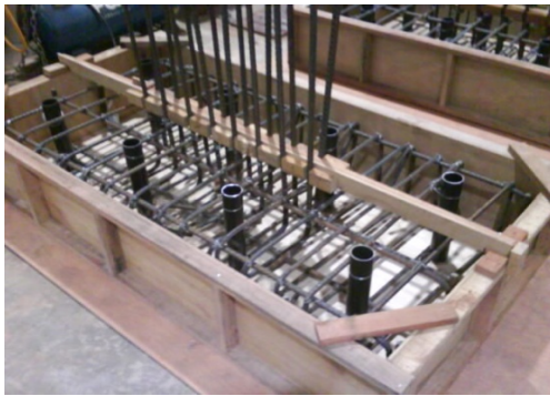
Fig. 4. Preparation of foundation beam
