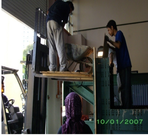
Fig. 6. Pouring concrete into mould
