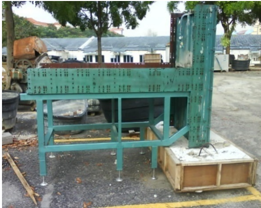
Fig. 8. Set-up of mould on foundation beam
