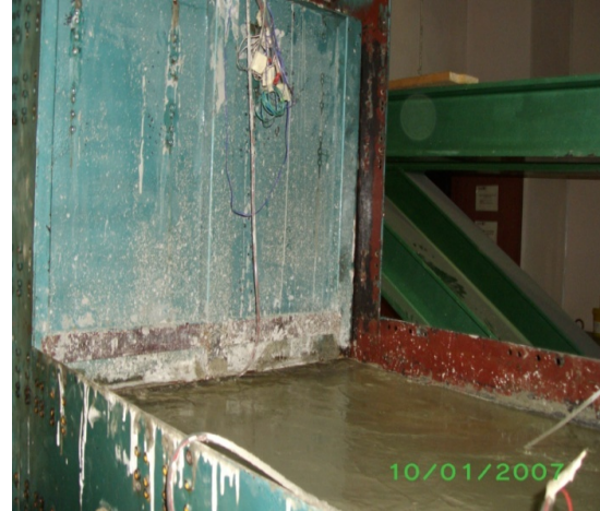
Fig. 7. Smoothing the concrete surface
