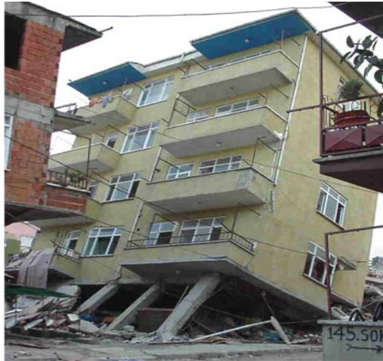
Fig.1 Soft story collapse of a building
