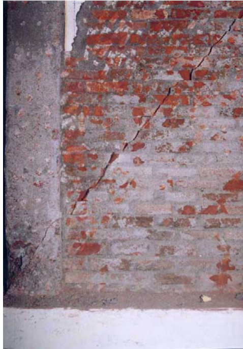
Fig. 6. Close up view of the crack after the plaster is chipped off.
