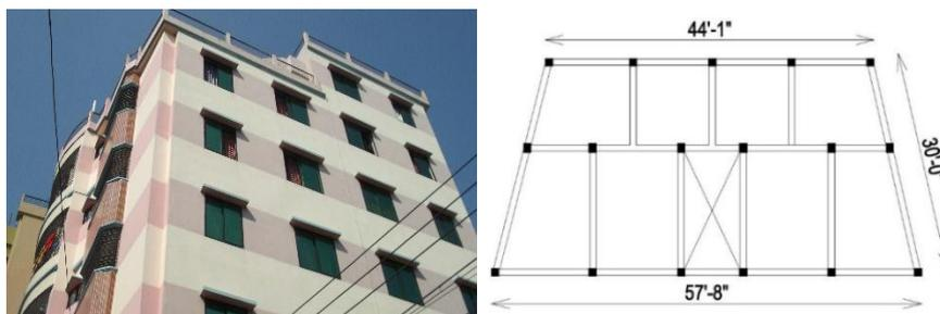
Fig. 4. (a) Prospective view of the index building; (b) typical floor plan.
