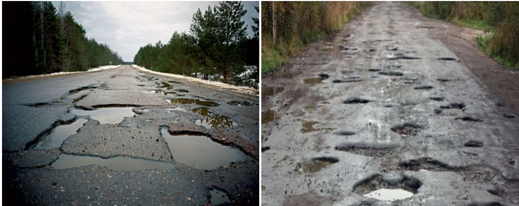
Fig. 1. Problem of flexible pavement for water logging
