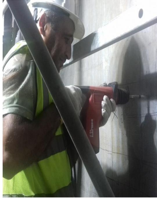
Fig. 5(b). Drilling of 48 mm hole for placing Anchor.
