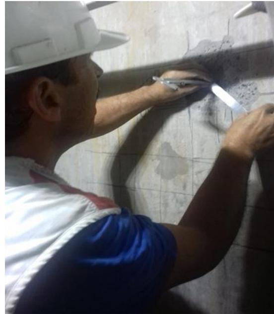
Fig. 9(b). Measuring the length of destruction.
