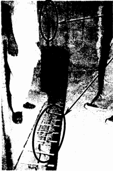
Fig 2a. Cracks and separated reinforcements of underpass W17
